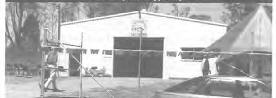
The new processing facility.
