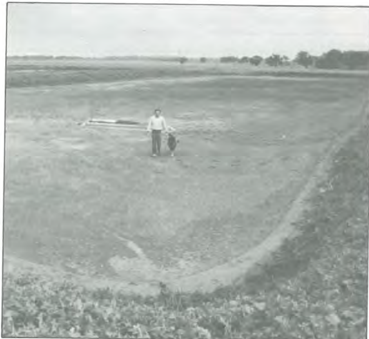
One of the fry ponds. The small concrete raceway houses fill and outlet pipes, and also is the collection point when fry are removed from the pond for sale.
